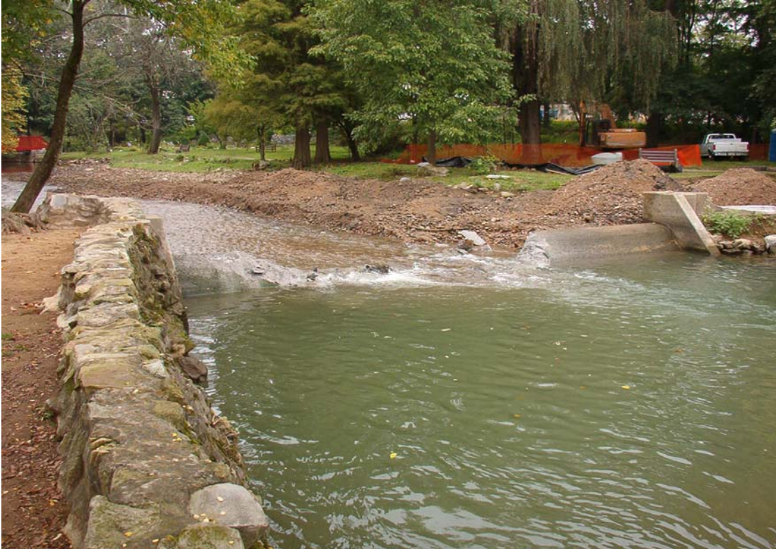
Photo 4. Reading Public Museum upper dam removal. September 2004
