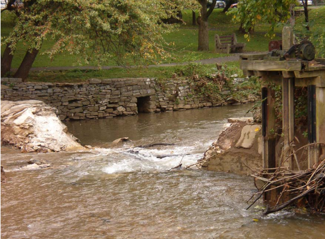
Photo 3. Reading Public Museum lower dam removal. September 2004.
