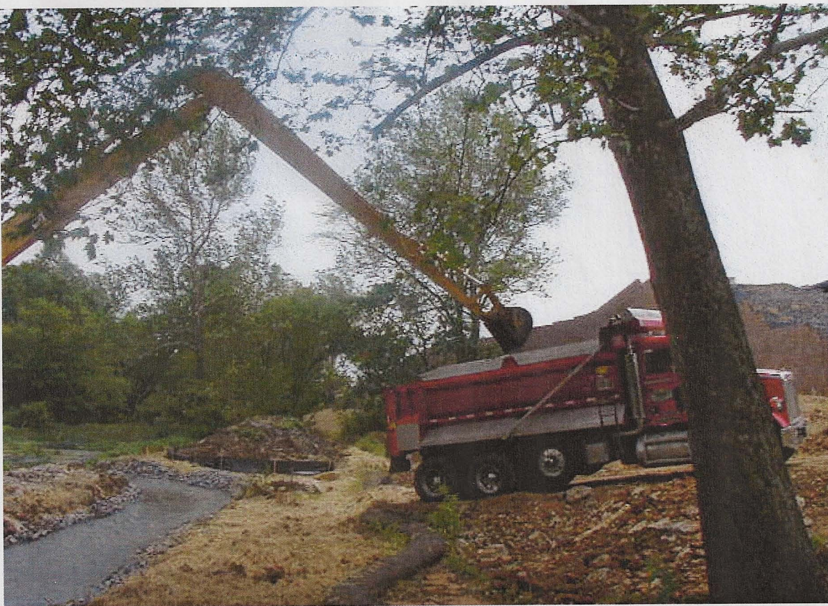
June 19, 2006 – Placing excavated sediment into trucks for disposal
