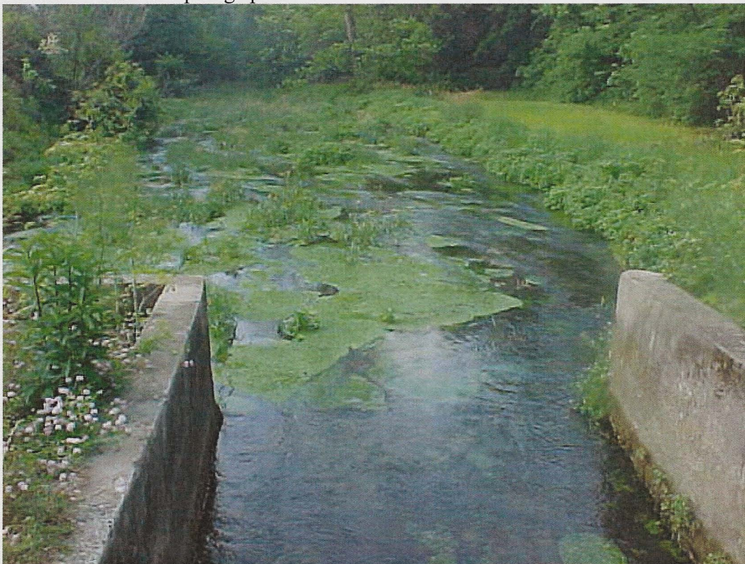
Picture 2 – reservoir and upstream view of dam
