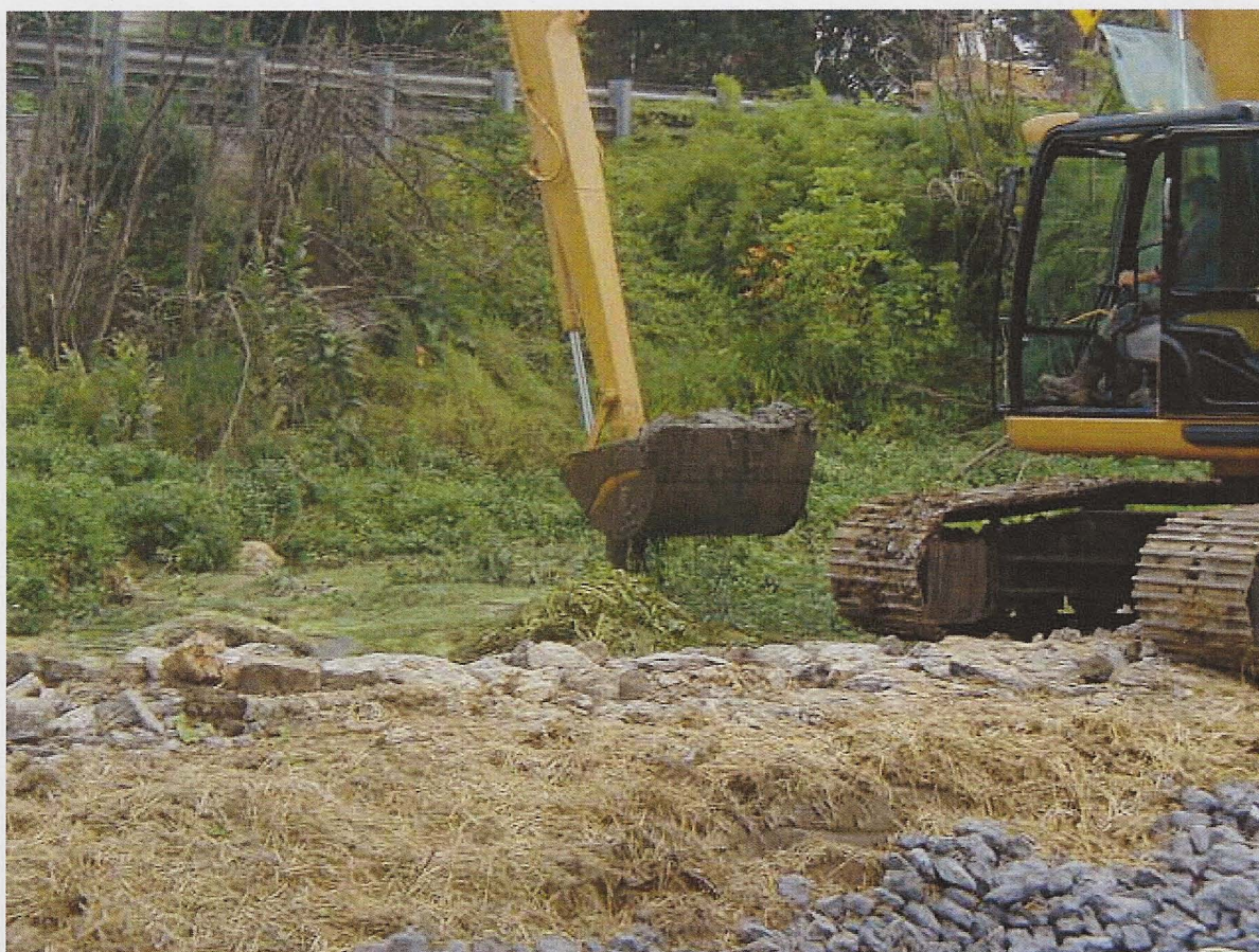
June 19, 2006 - Excavation of impounded sediment
