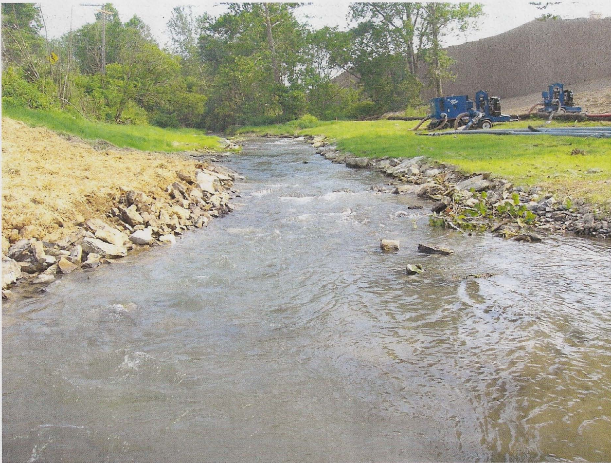
July 26, 2006 – Completed project
