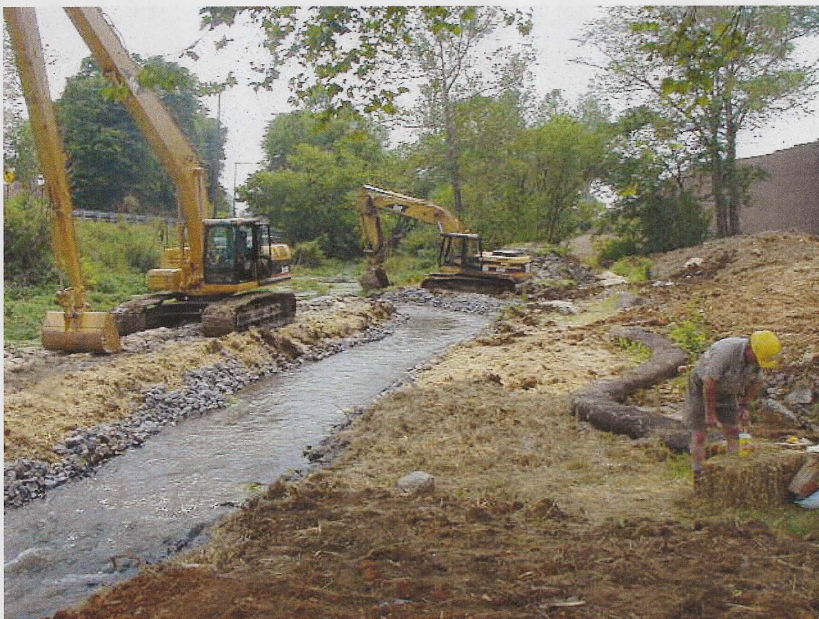
June 19, 2006 - Placing flow into bypass channel. Turbidity - 32 - 62 NTU
