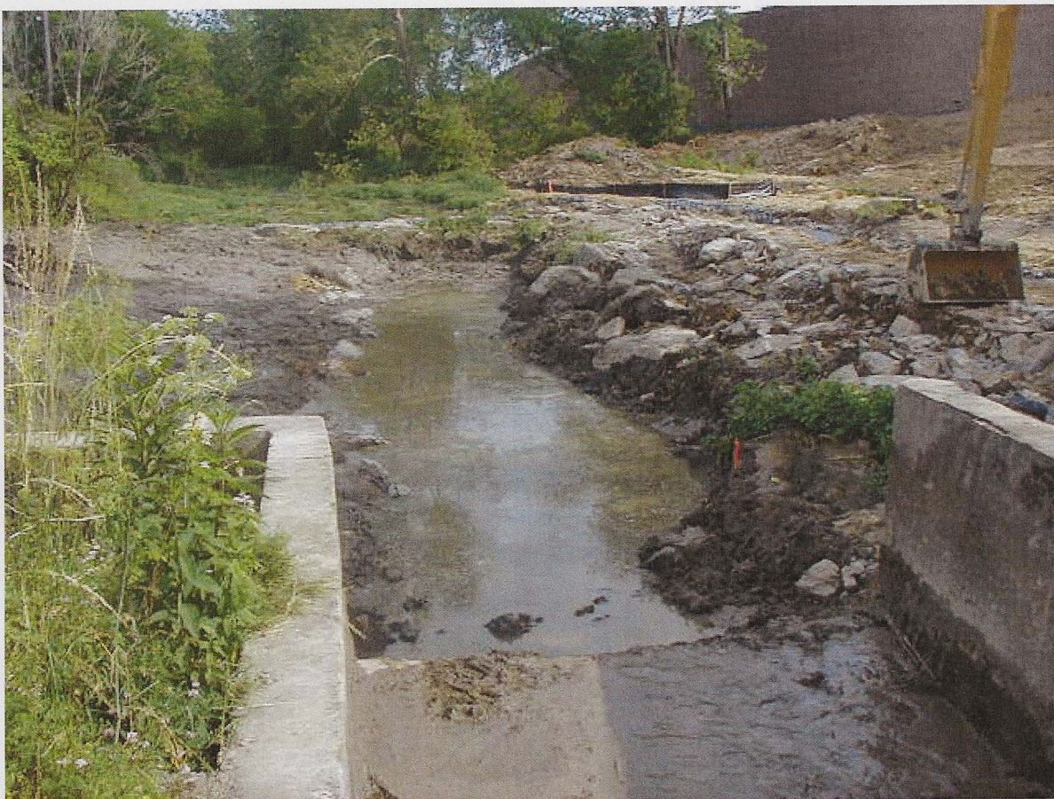
June 28, 2006 – Returning flow to permanent channel – turbidity 78 – 470 NTU
