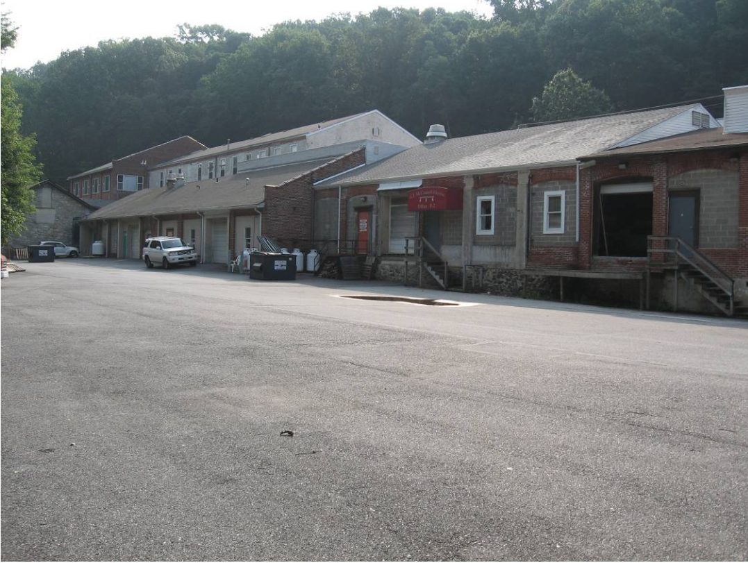
Photo 5. Businesses adjacent to Unnamed dam that are impacted by flooding.
