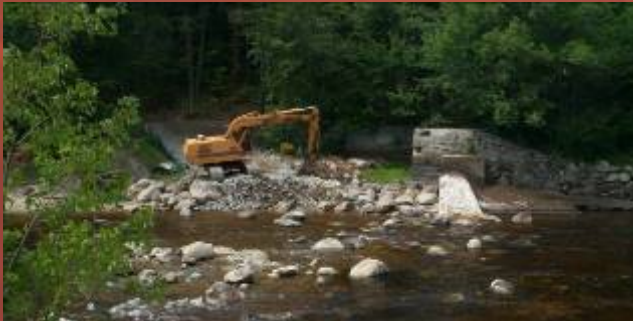
Removal of dam in June 2004
