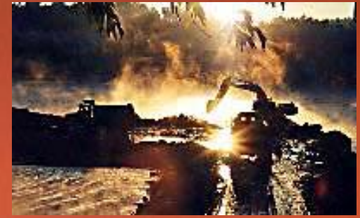
Edwards Dam Removal, ME
