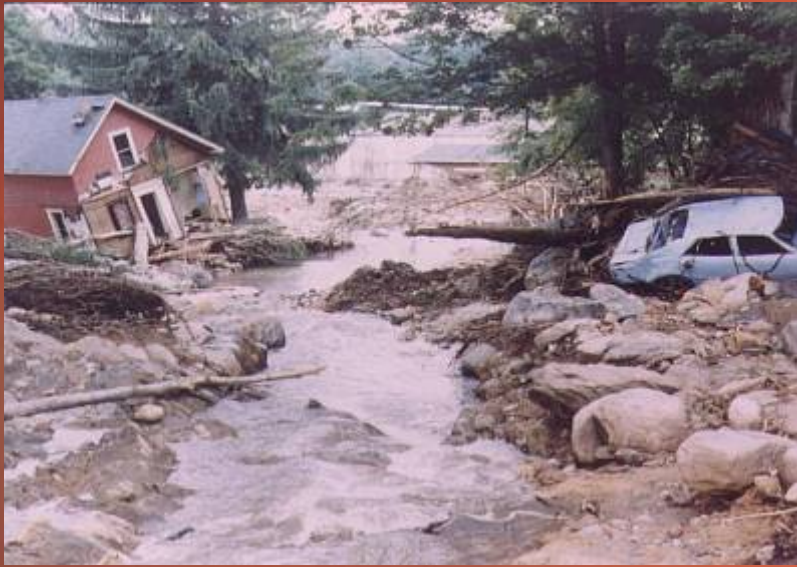
Connecticut Dam Failure - Source: Jim MacBroom
