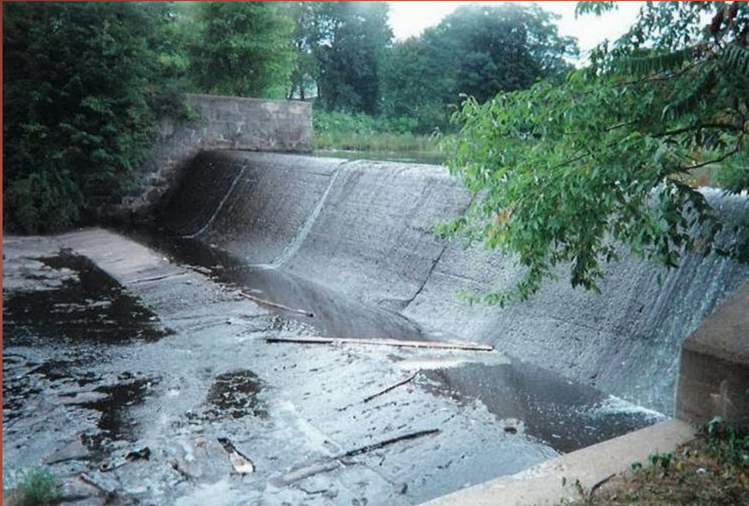
Brass Company Dam – West Branch Naugatuck River – Torrington, CT
