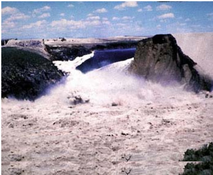
Teton Dam failure, ID, 1976
