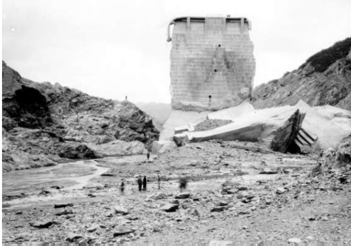
St. Francis Dam failure, CA, 1928
