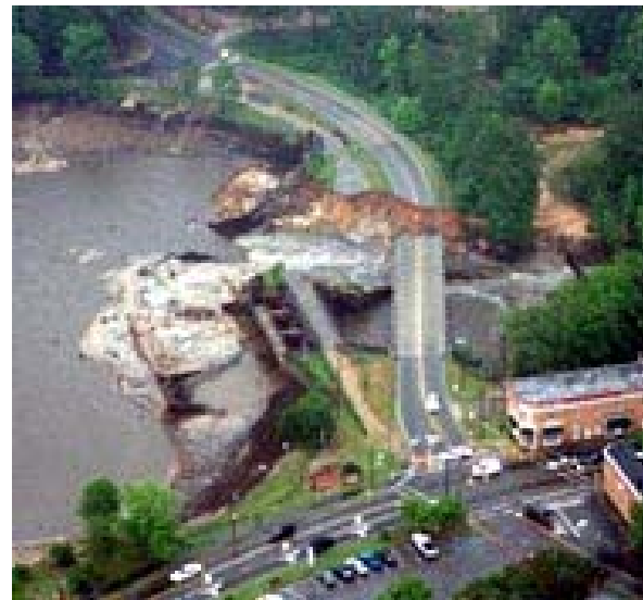
Rockfish Creek dam failure, NC, 2003
