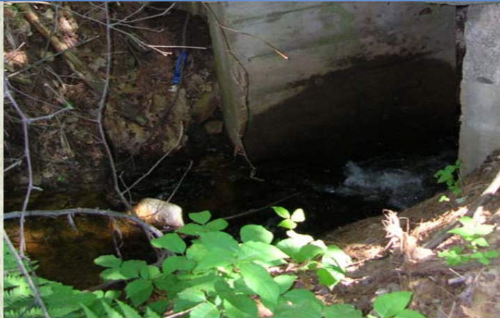
Whitehouse Road Culvert
