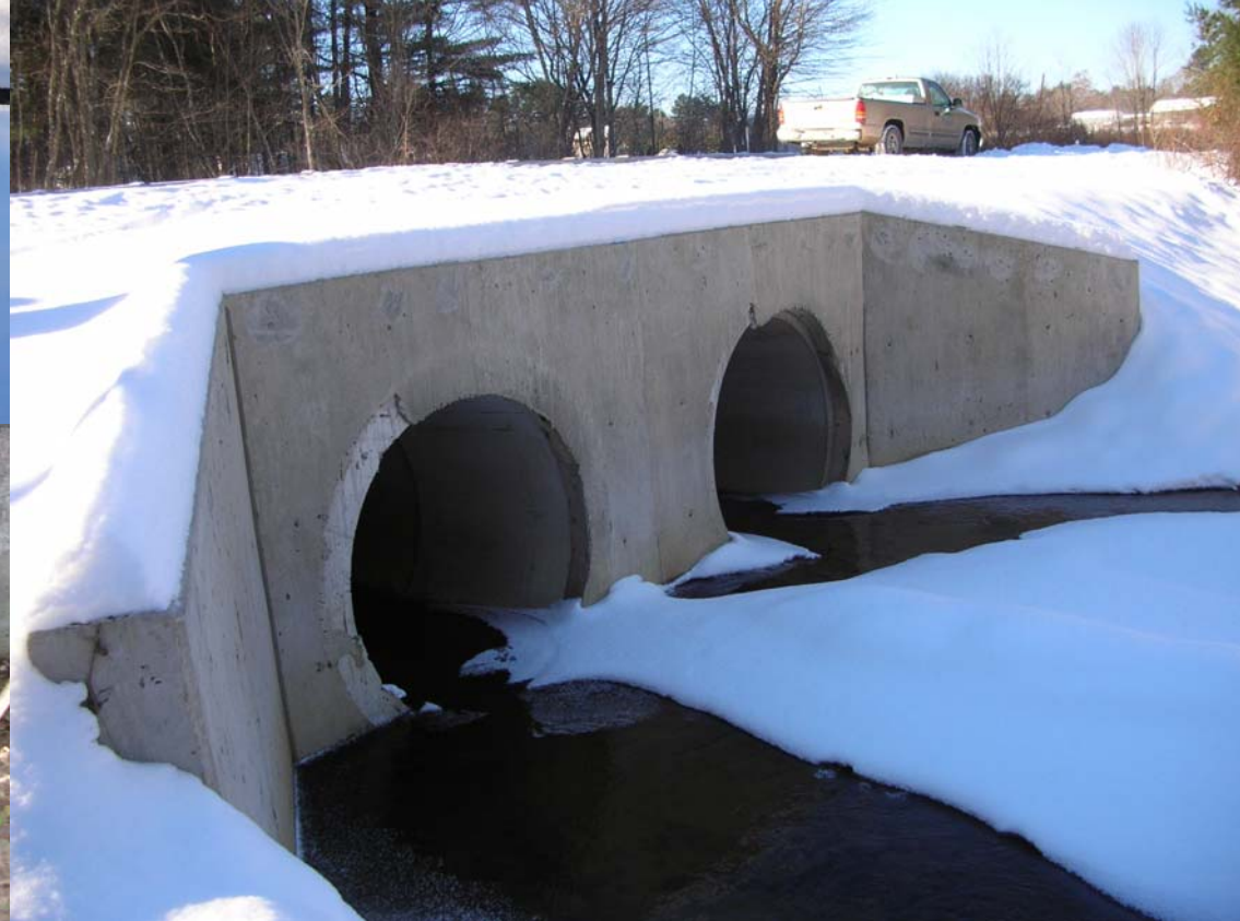
Old Dover Road Culvert
