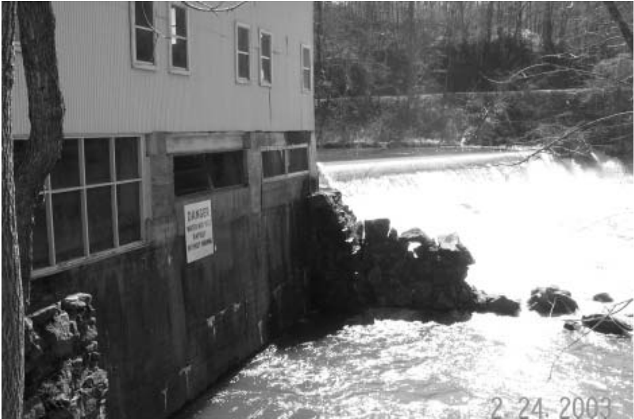
Photograph 1 Dillsboro dam and powerhouse tailrace, note high flows from recent rainfall.
