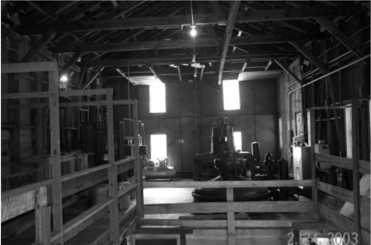
Photograph 3 Dillsboro powerhouse interior, both units visible.
