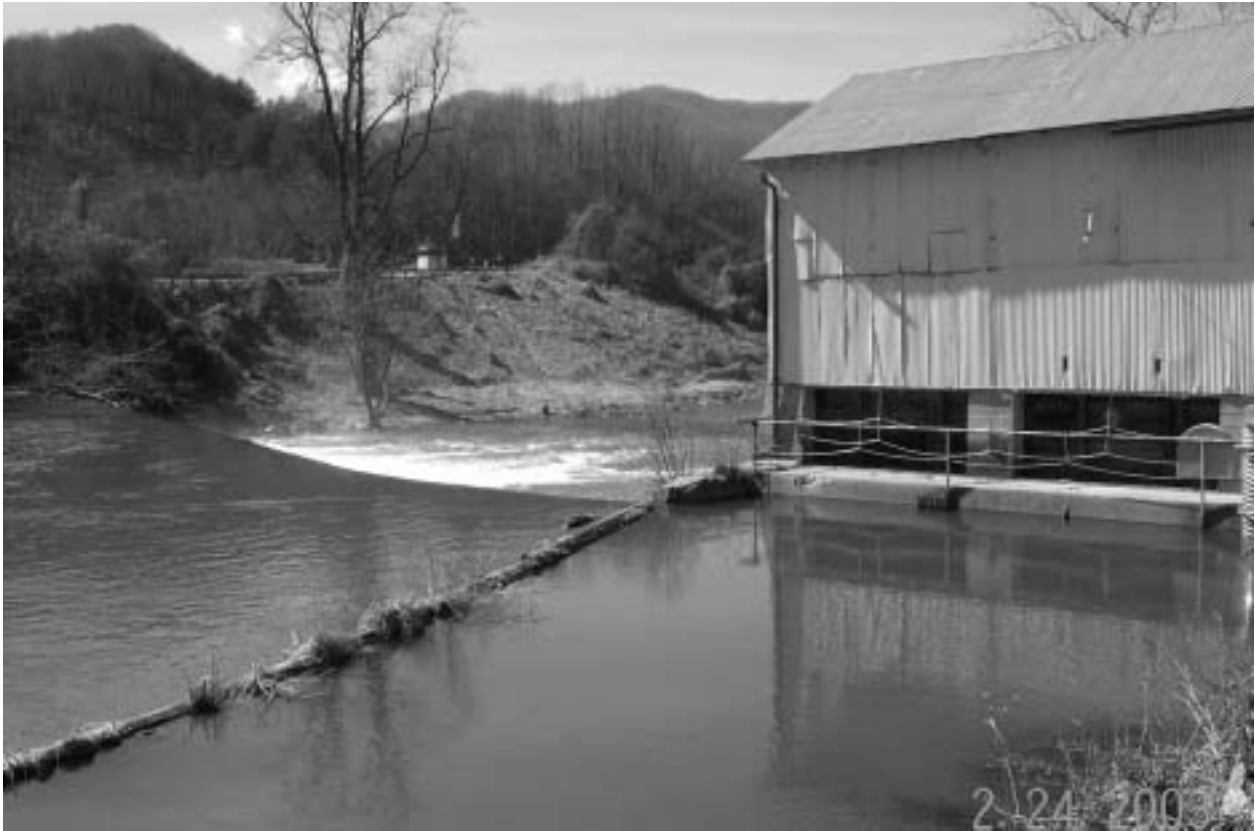
Photograph 2 Upstream side of Dillsboro dam and powerhouse as seen from the right bank.
