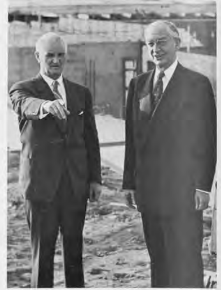
Watkins showing Sproul construction progress.
