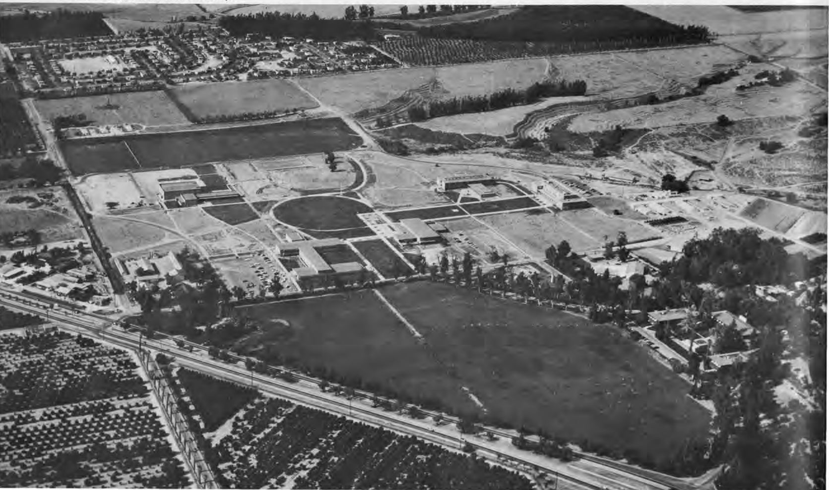
A view of the original five buildings taken in 1955. Left to right: Physical Education, Social Science and Humanities, Library, Physical Sciences, Webber Hall (then the Life Sciences).
