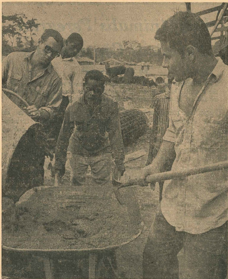
Peace Corps volunteers Gerald Underdal (left) and David Torrice work on a school construction project in Gabon, West Africa. They are among several volunteers assigned to the school building program in the French speaking country. Local self-help labor is used in the construction while Volunteers supply technical expertise and supervision.
