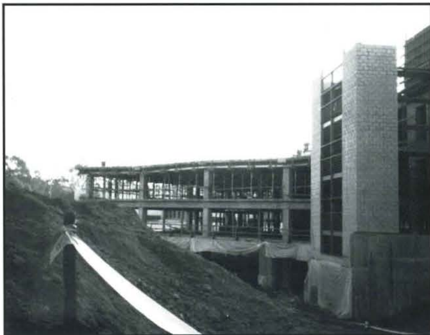
After over a year of construction, UCI's second parking structure will be ready to accommodate 7 cars near Bren Events Center.
