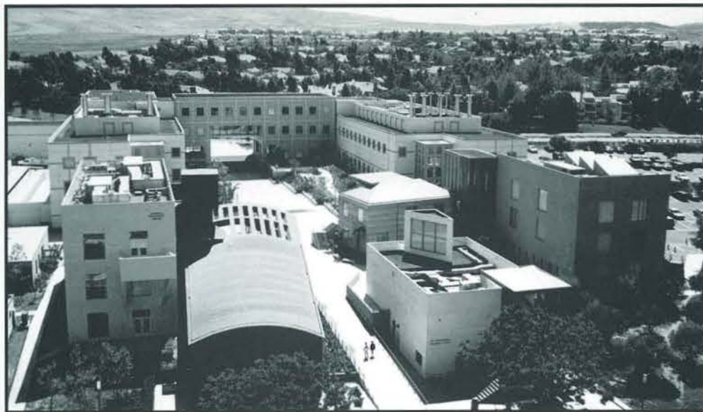
LEFT: Several structural changes greeted the students at the start of the 1994-1995 school year, including the new Engineering Gateway area.
