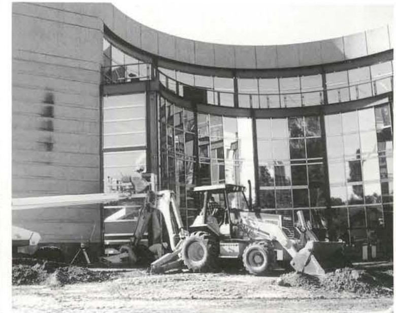
Construction takes place on a hot summer day for the brand new natural sciences building, for both physical and biological sciences.
