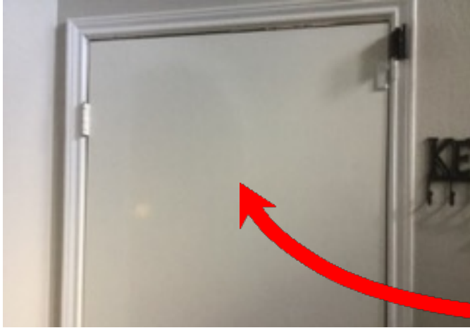
Garage Passage Door Peephole No peephole
