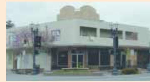
One of the many projects being funded is the rehabilitation of eight apartments on the corner of Texas and Jackson Streets.
