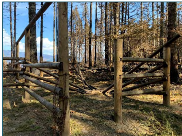
Photo 8. Horse Camp corral damage
