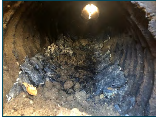
Photo 5. Burned out culvert
