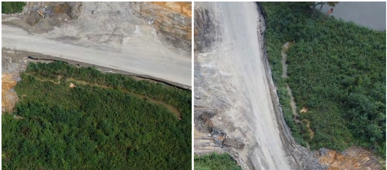
Black silt fence along mining road seems to be completely overrun by sediment and rock, allowing muddy water, sediment and debris to enter W-3 (left photo) before it goes under apparent fill and mining road and into the protected stream buffer for S-5. Note visible contrast in stream color in left picture (water is muddier adjacent to downed silt fence). The overrun silt fence is barely visible in the picture at right, which appears to show W-3 flowing down from P-3 (at top of picture) until it hits the apparent unauthorized fill area.
