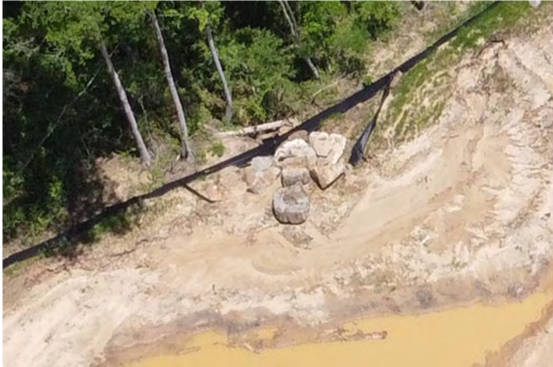
Silt fence seemingly not properly installed near Sediment Basin 005, allowing water & sediment to flow over & under silt fence. (5/7/21)
