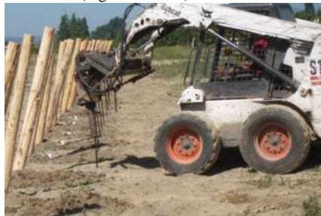
**Figure 8.** Drilling in post anchors
