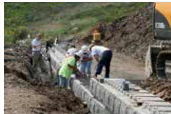
INSTALLING GEOGRID HORIZONTALLY
