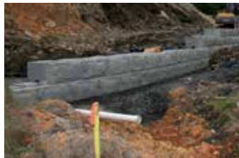
INSTALLING THE FIRST COURSE
