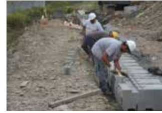
CLEANING DEBRIS OFF UNITS
