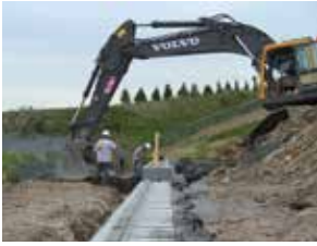
INSTALLING THE FIRST COURSE
