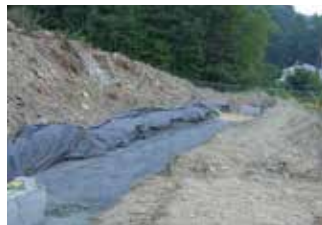
LEVELING PAD AFTER COMPACTION
