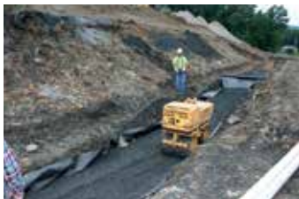
GEOTEXTILE AND COMPACTION
