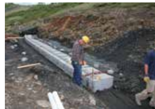
LEVELING EACH UNIT
