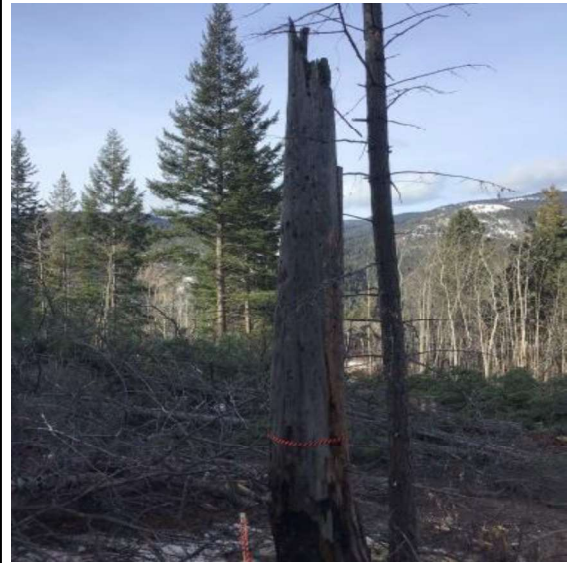
Tree clearing for transmission line.
