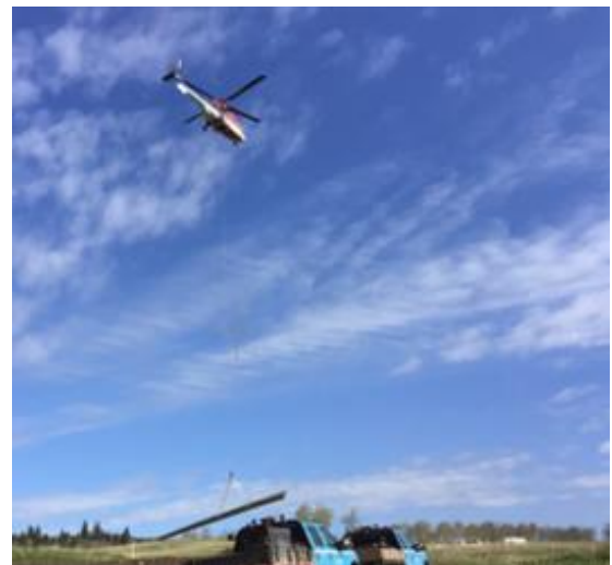
Aerial operations transporting transmission poles.
