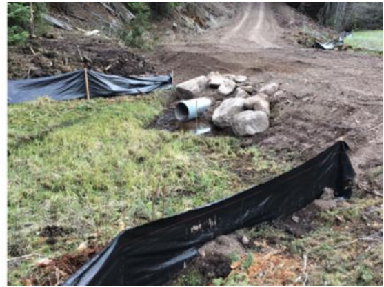
Sediment fences installed throughout site during the spring thaw.
