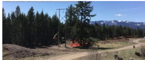
Tree removal near transmission line.
