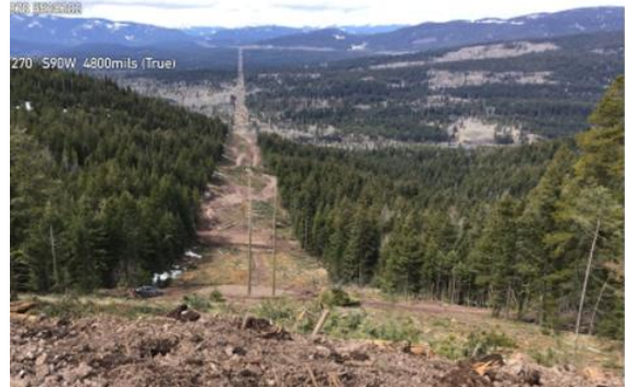
Existing cleared transmission line.
