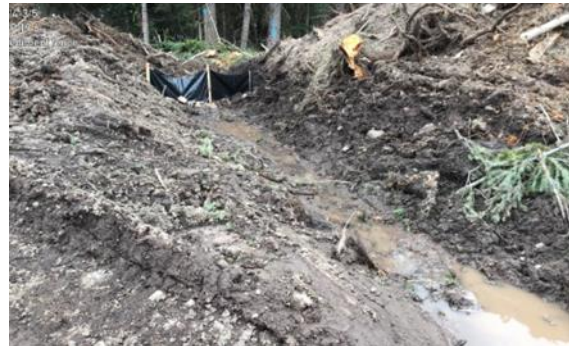
Sediment fences installed throughout site during the spring thaw.
