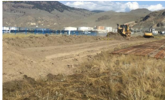
Topsoil stripping on the KUA ROW.
