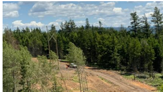
Contractor re-seeding along transmission line.
