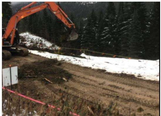
Forest debris used for topsoil cover as an erosion control measure.
