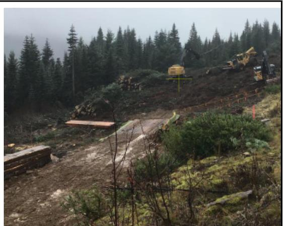
Timber placed along the right-of-way to be processed and bucked for transport at KP 990.
