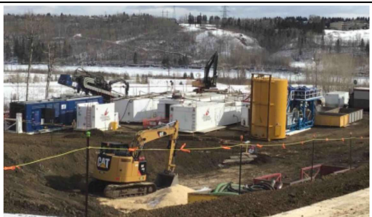
North Saskatchewan River HDD west side.
