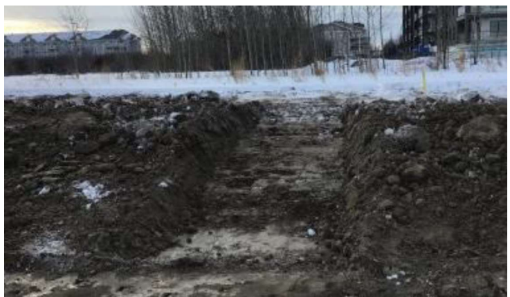
Drainage paths excavated to maintain drainage and capture sediment
