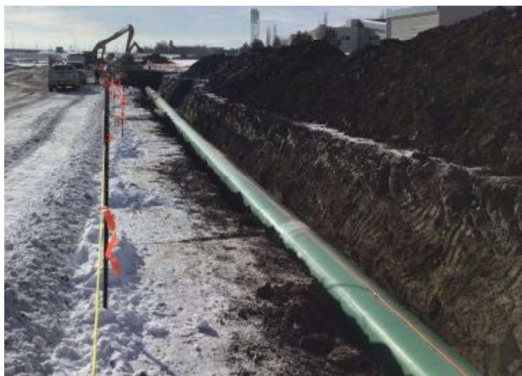
Installed pipe with fibre-optic leak detection system.
