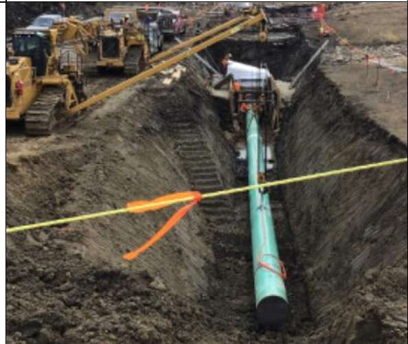
Welding mainline and water by-pass around trench.
