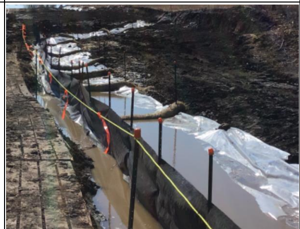
Water filtration and matting placed to preserve top soil consistency.
