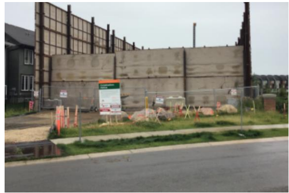
Noise barrier near a residential community.
