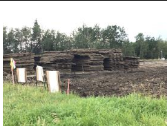
Cleanup on right-of-way, including removal of rig mats.
