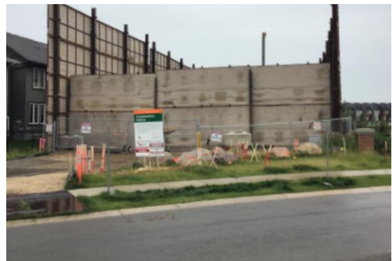
Noise barrier near a residential community.
