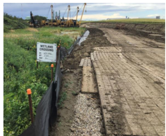
Silt fencing near a wetland.
