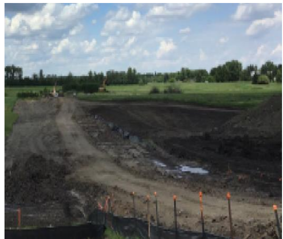
Cleanup on right-of-way.
