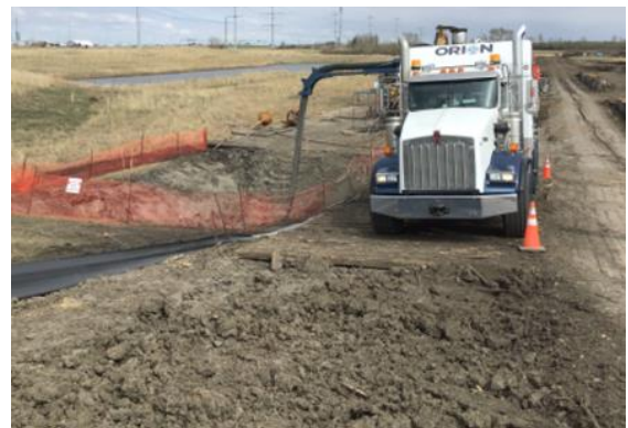
Hydrovac excavation during the drilling activities.
