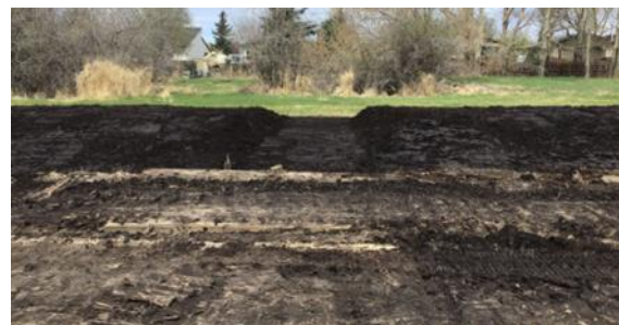
Drainage paths excavated to maintain drainage and capture sediment.
