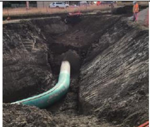
Pipe during backfilling.
