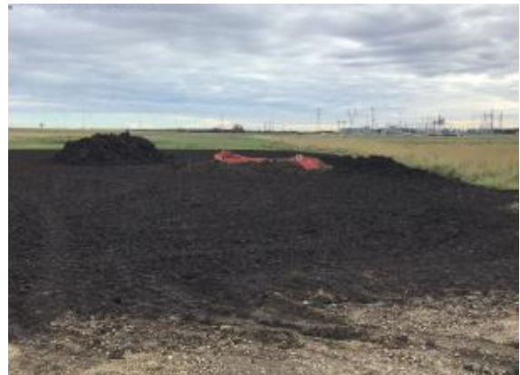
Topsoil reclamation nearly complete.
