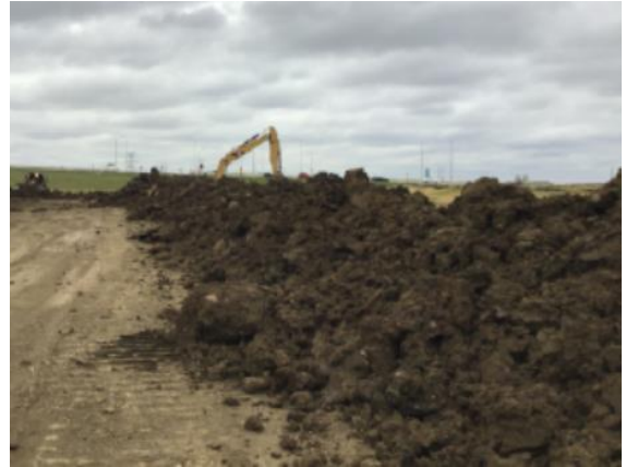
Return and compaction of roach pile.
