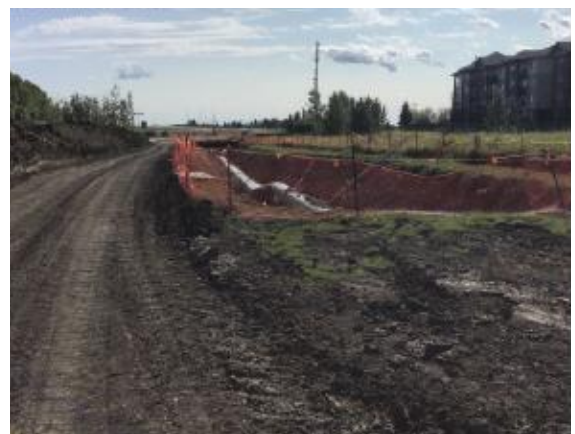
Ensuring excavation is properly signed and fenced.
