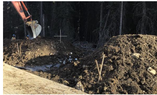
Topsoil being separated before covering.
