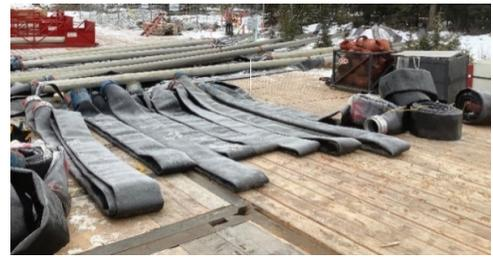
Dewatering pipe being stored in preparation for pipe replacement work.
