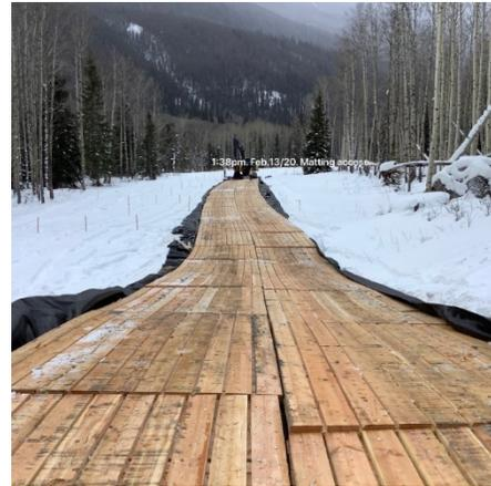
Protective matting made of Douglas Fir placed on an access point to the Project right-of-way.
