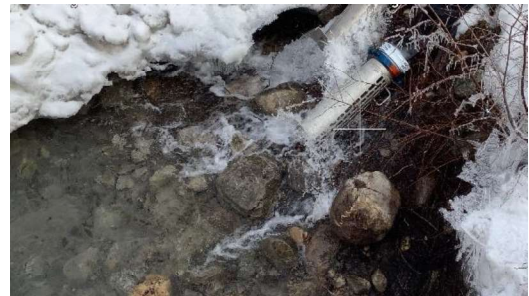
Water defuser used to redirect water during instream work.
