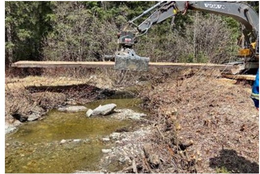
Bridge removal after instream works complete.
