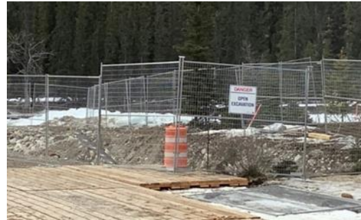
Fence installed to keep wildlife from entering construction area.
