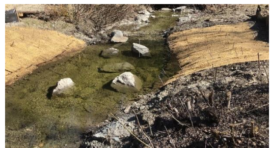
Restoration of watercourse bank using willow staking and instream boulder replacement.
