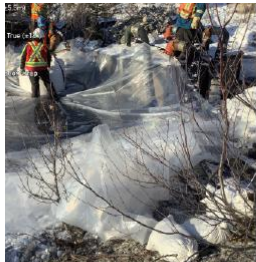
Vine Creek stream isolation, water pumping.
