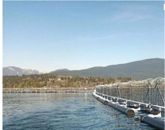
Bird landing deterrents on the marine construction safety boom.
