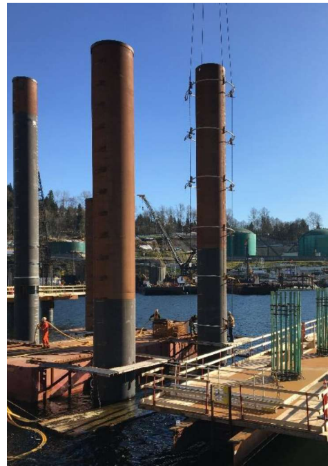
Bubble curtain being installed on an offshore pile.
