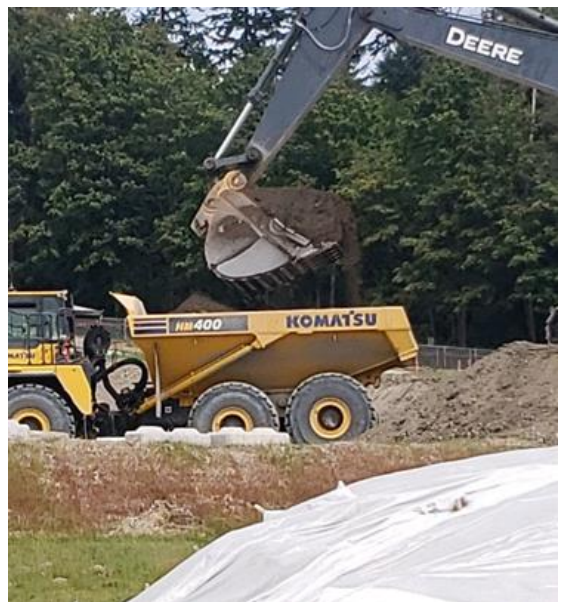
Truck being loaded with soil for removal from site.
