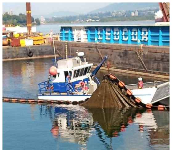
WMT turbidity curtain being cleaned.
