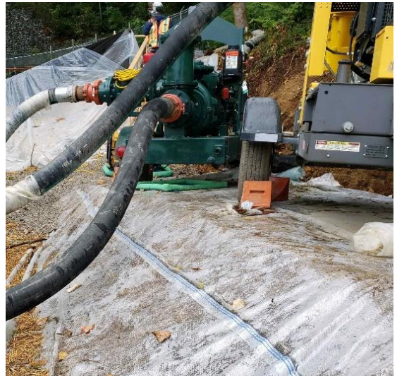
Diversion pumps at Eagle Creek at Burnaby Terminal.
