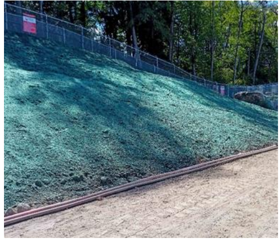
Hydroseeding (ESC) at WMT.
