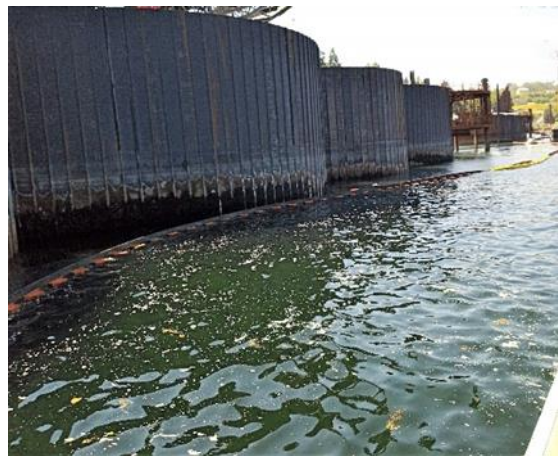
Turbidity curtain surrounding the foreshore expansion at WMT.
