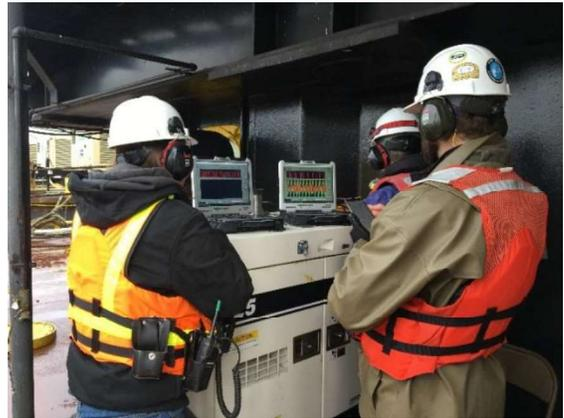
Environmental monitors and Contractor Superintendent monitoring underwater noise levels during offshore impact pile driving.
