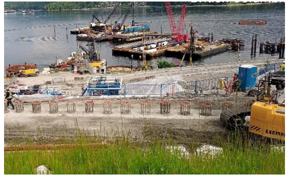
Secant wall construction at WMT.
