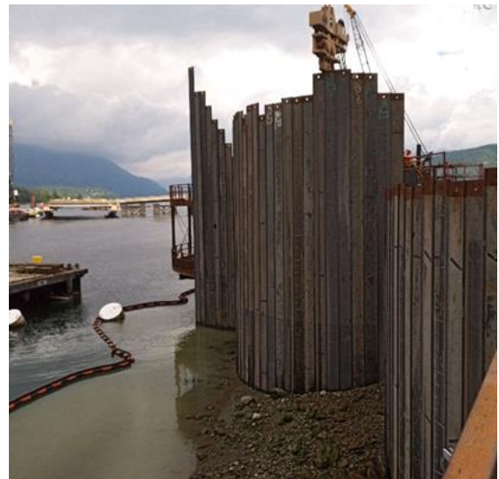
Sheet pile cells, part of shoreline construction works at WMT.
