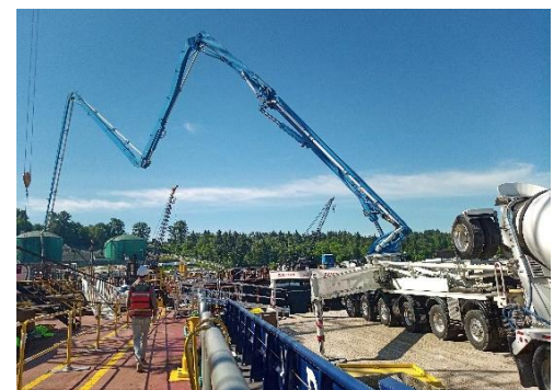
Cement truck pouring into dolphin jacket leg.
