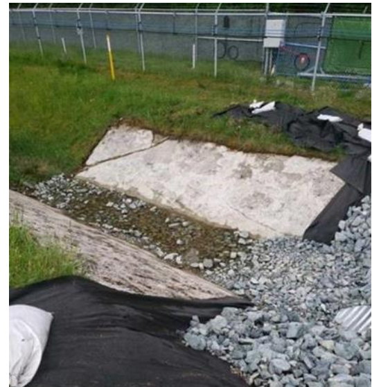
Drainage canal at Burnaby Terminal.
