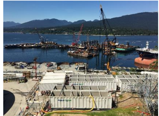
Offshore marine work area and foreshore construction.
