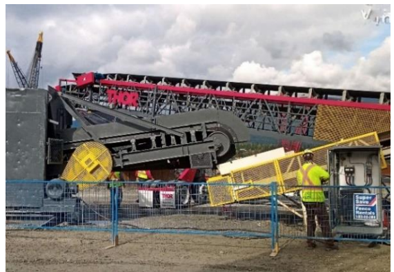
Conveyor taking cured grout spoils material to barge for offsite disposal.
