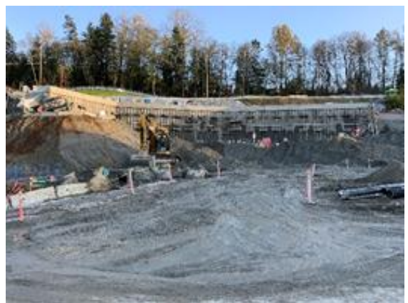
Construction of the Burnaby Mountain Tunnel Portal at WMT.
