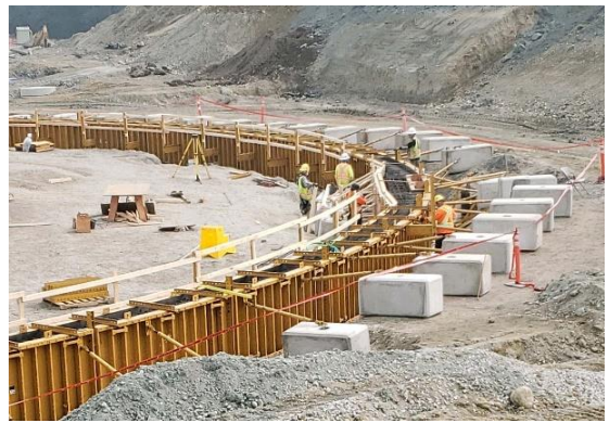
Tank foundation frame prior to concrete pour.
