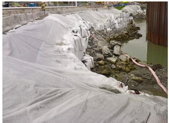
Polyethylene sheeting used as an ESC measure along the shoreline at WMT
