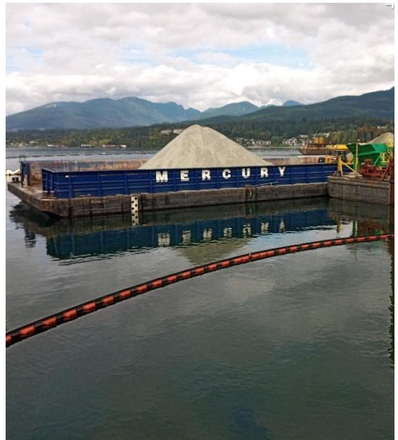
Turbidity curtain at the WMT foreshore.
