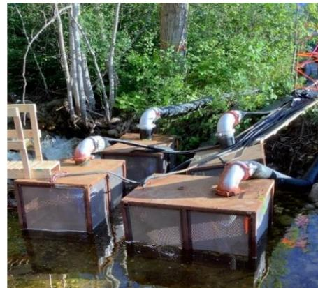
Upstream diversion pumps used in conjunction with an Aqua Dam isolation to successfully divert and maintain watercourse flow
