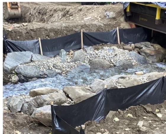
Silt fence set up for sediment control.
