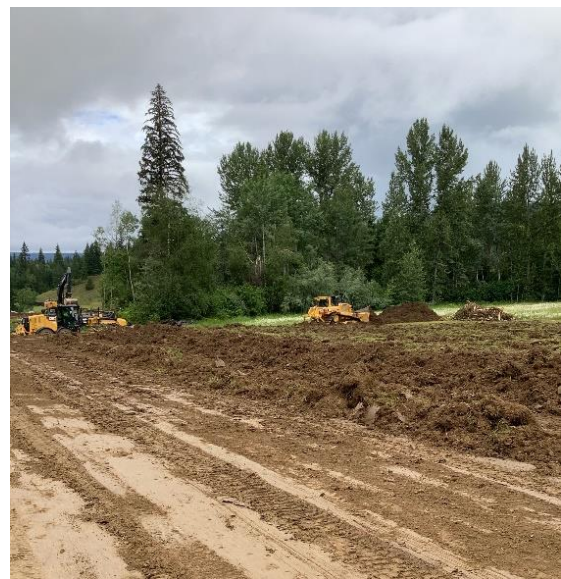
Topsoil being stripped.
