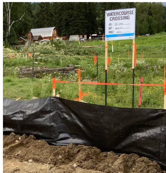
Silt fence sediment control and signage in place.
