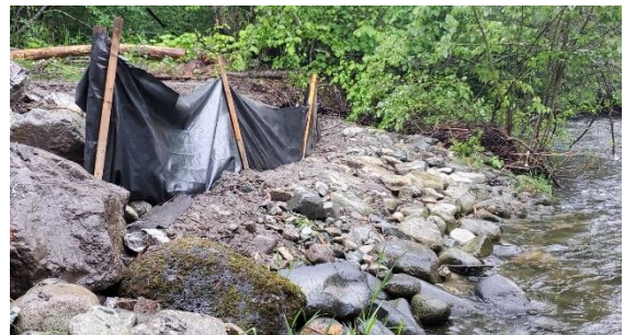
Bridge replacement silt fence sediment control in place.
