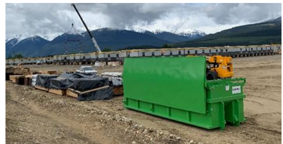
Waste sorting at Valemount Camp construction site.
