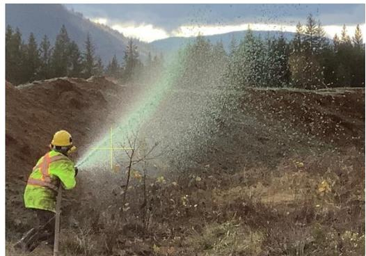
Hydroseeding of topsoil near access road Shoefly 23.
