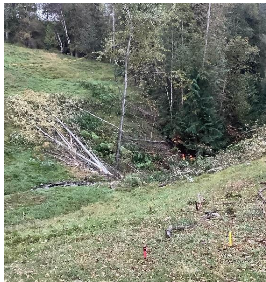
Clearing of trees near Peavine Creek.
