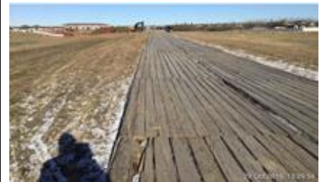
Matting on the Project right-of way
