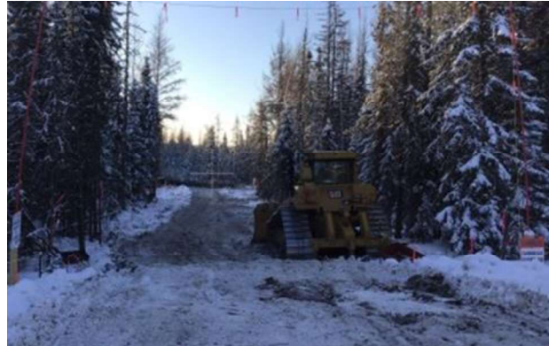
Monitoring clearing for access to right-of-way
